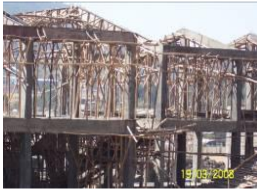
Figure 4. Eucalypt woods for transmission poles and construction poles and posts in Ethiopia (Photo by Mulugeta Lemenih)
